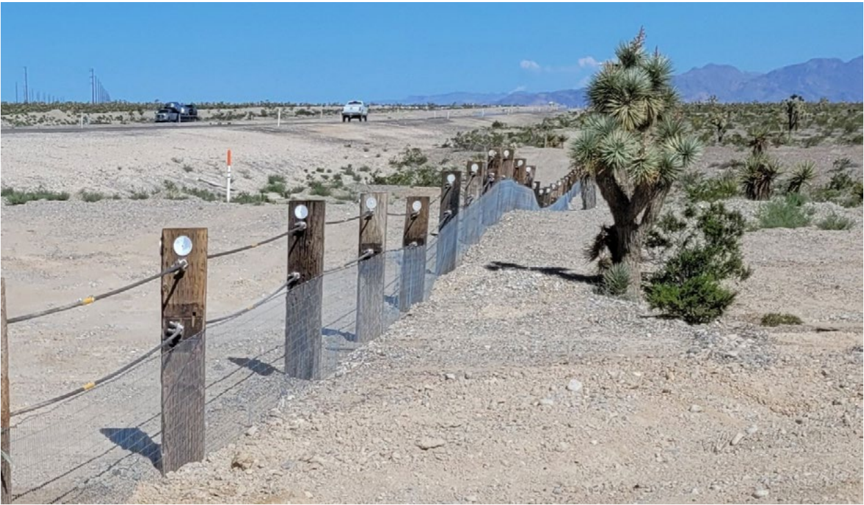
Completed combination post and cable tortoise fencing along US95 and Tule Springs Fossil Beds National Monument.
