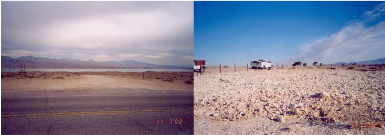
The entrance to Approved Road 108 from Northshore Road in 2002 prior to decommissioning and ripping treatments (left) and four days later after decommissioning, ripping, and fencing was installed (right). Photograph provided by Lake Mead National Recreation Area archives.
