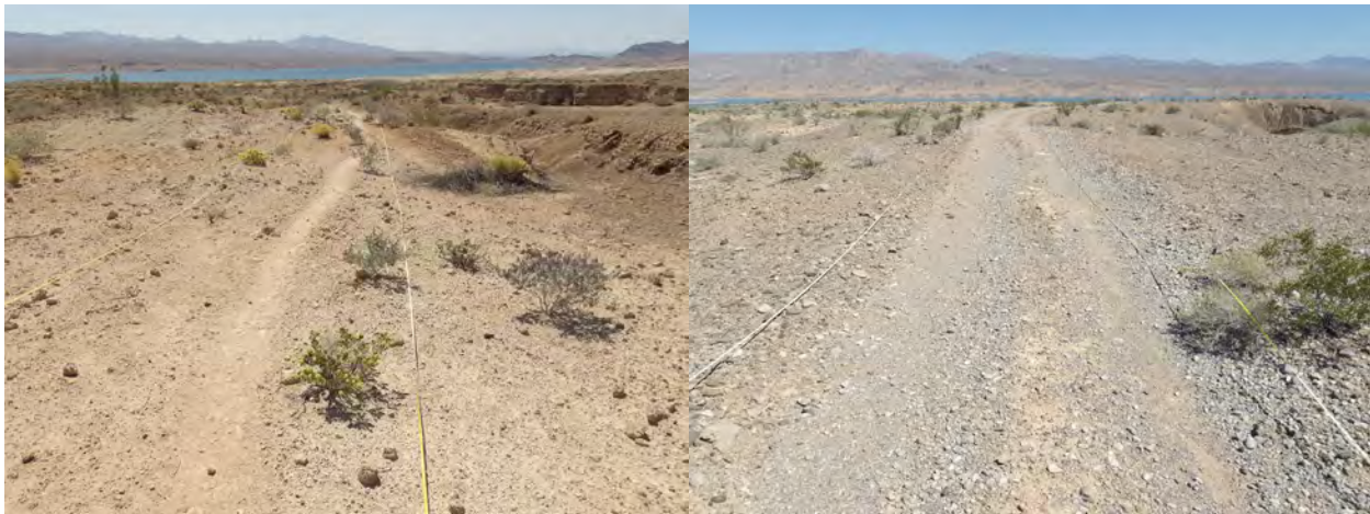
Example restoration plot that received ripping (left) and a plot on the same decommissioned road but that was unripped (right), Road 108 Soil Ripping project. There is a narrow trail shown in the center of both photos, as the road was closed to vehicles and converted pedestrian access only via the trail. Photos taken in March 2024 by UNLV staff (plots RIP06, NRIP02).
