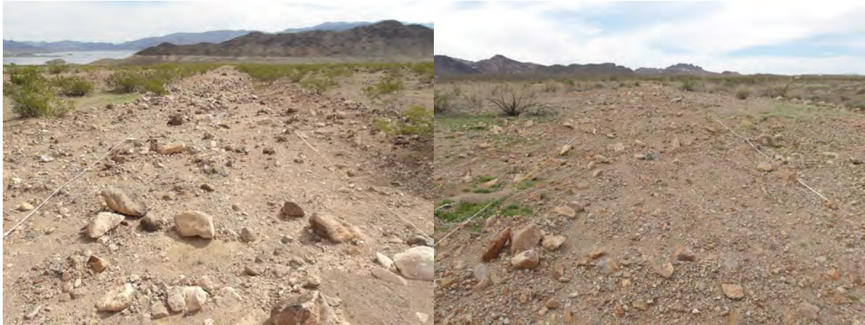
Example restoration plot receiving soil ripping and outplanting (left photo) and a control plot (right) both on the same decommissioned road, SNWA Endcaps Planting project. Photos taken in March 2024 by UNLV staff (plots SNWA1P, 2C).
