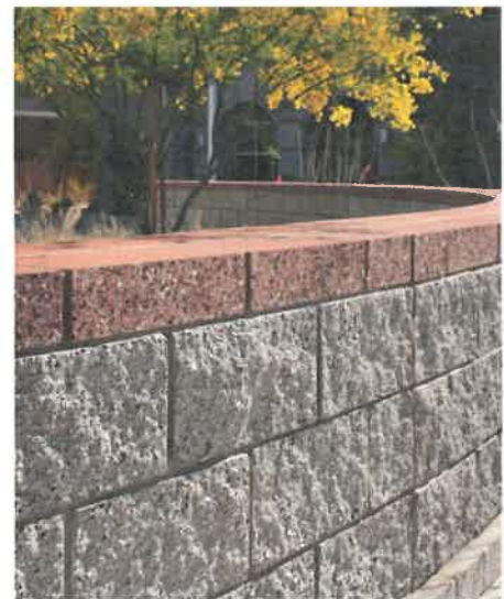
An integral colored CMU smooth finish cap on top of a gray split face wall showing significant aggregate within the block. This style of gray block is acceptable.
