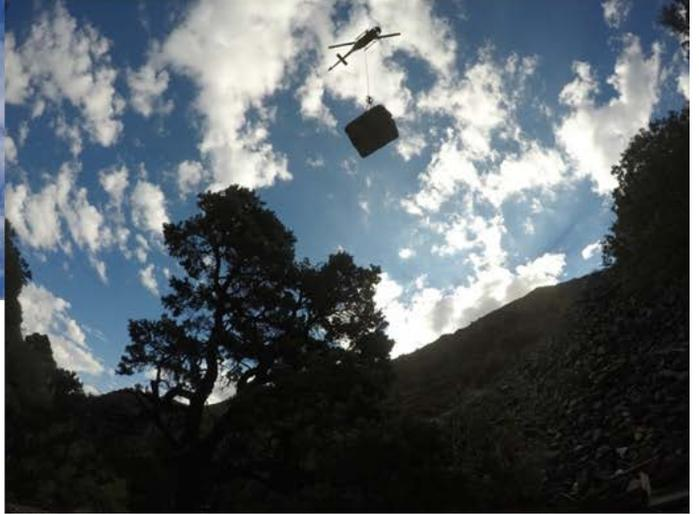
Left: Helicopter transporting a culvert using a super sack bag creating drag reducing spin during transport
