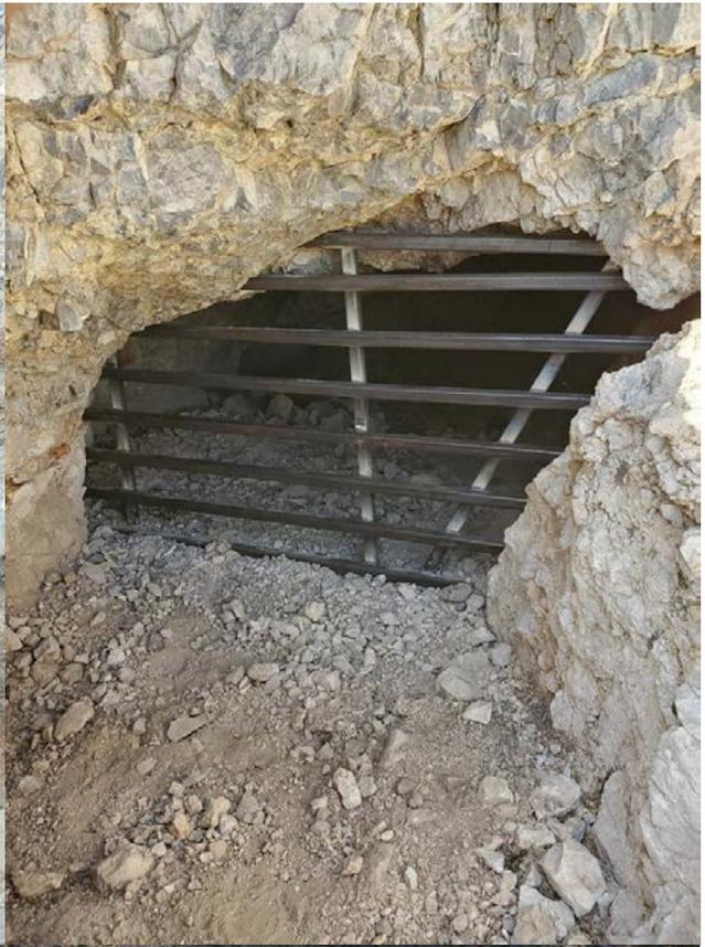
Two completed gates and a small materials landing zone for hazards at the Goodsprings project
