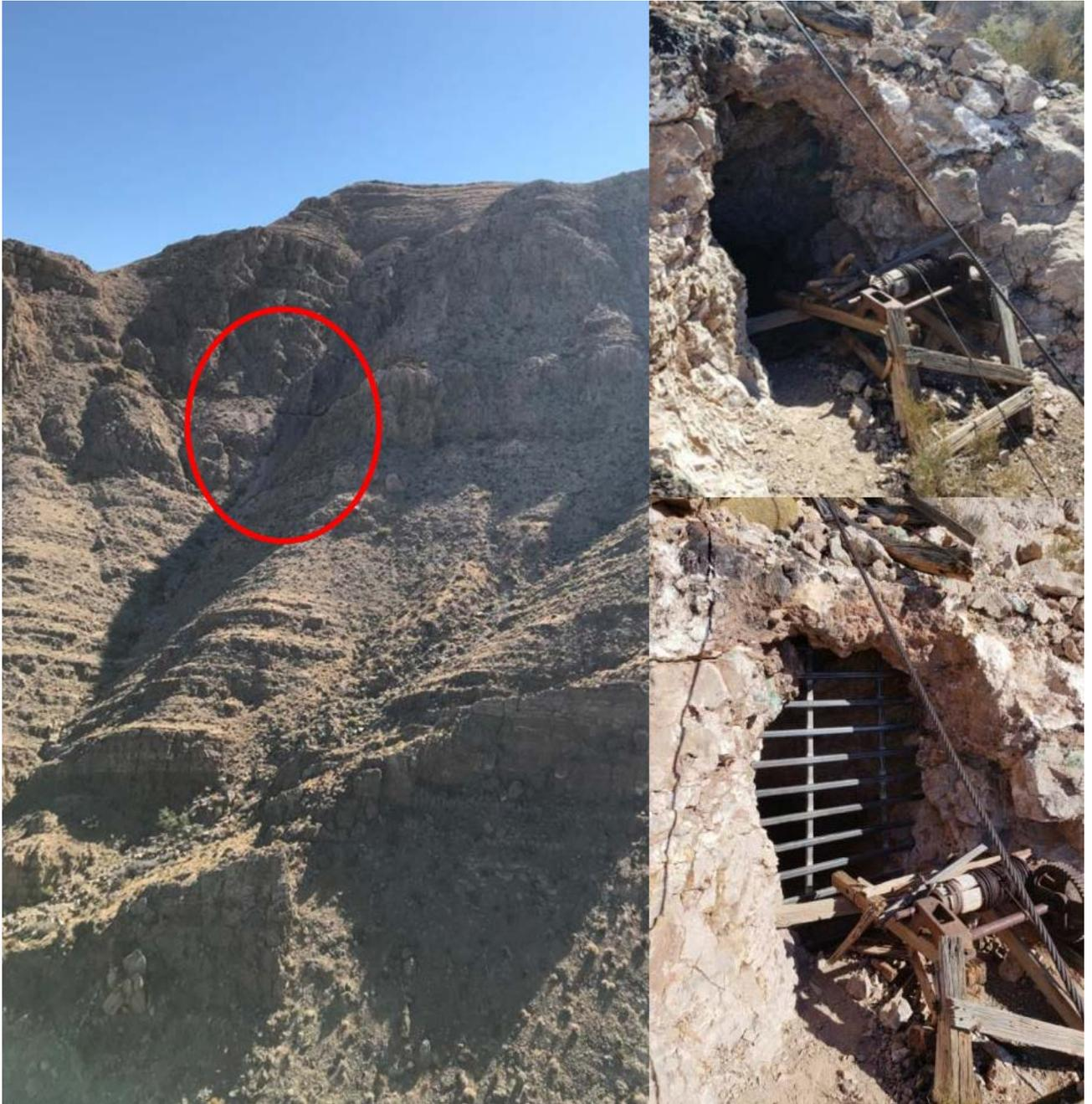
The Tramp Complex apart of the Gold Butte Project: although remote, an established unofficial hiking trail was used to hike personnel to the site after the materials were dropped off by the helicopter. The before and after photos on the right illustrates how EPS was able to construct a wildlife gate without impacting the cultural resources.
