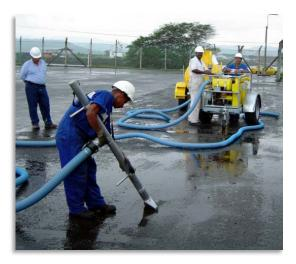
Vacuuming water from pressure washing activities is an effective way to keep waste water from entering the storm drain system.
